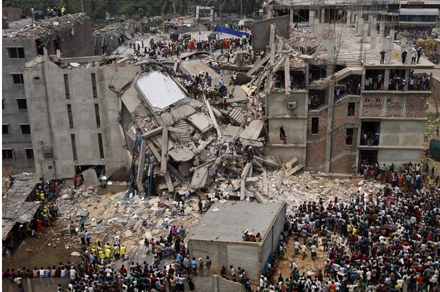
Figure 2. Aerial view of collapse.
